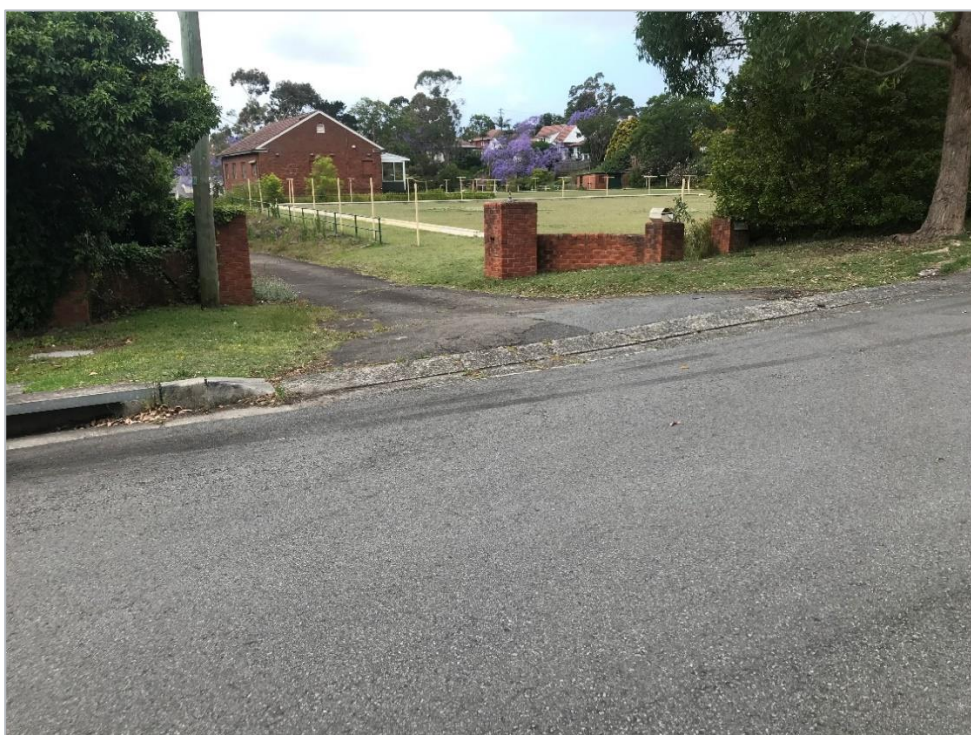
Figure 1-2 Site frontage and driveway to Warrane Road
